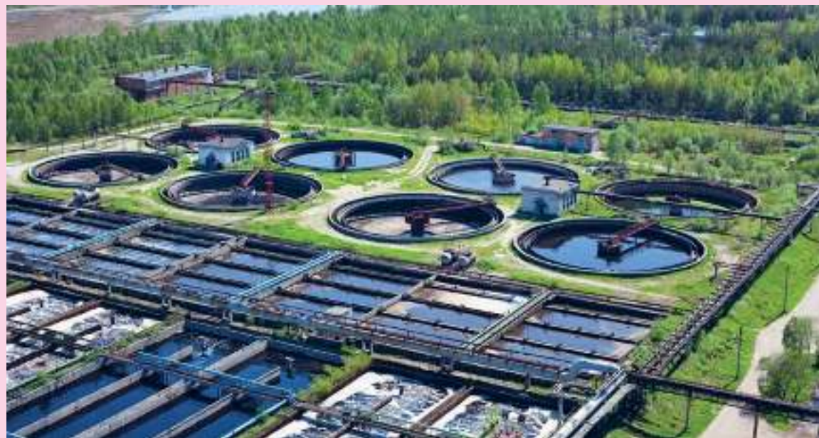
Sewage Treatment Plants
